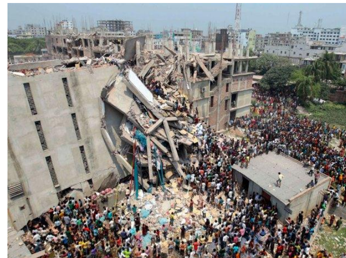
Building collapse, Bangladesh, 2013
